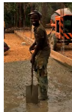
Francis Andoh (lead mason, foundations, columns and beams)
