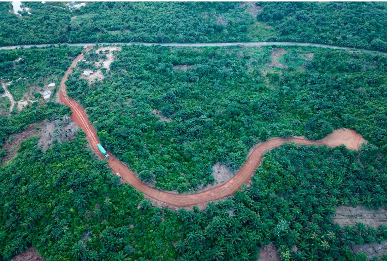
Drone image of the access road constructed in April 2019.
