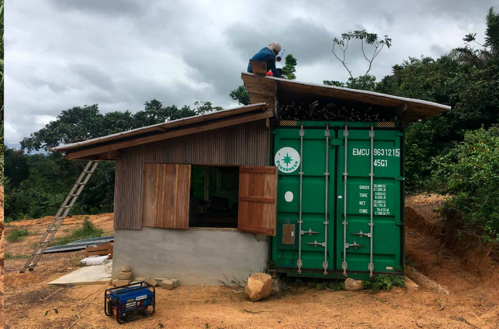
21 Replacement of the blue 2-kW gasoline generator (left) with solar power; the panels are located on the bamboo roof of the green container (right), which is also shown in the schematic diagram on page 19.
