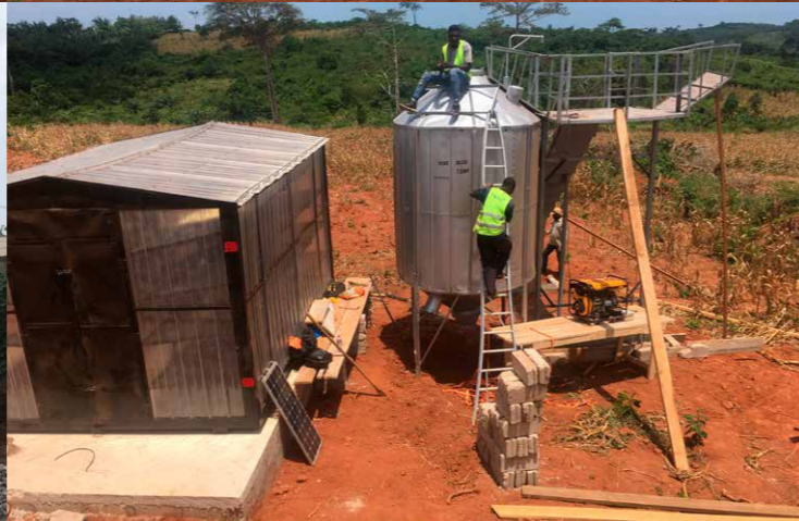
Impressions of the construction in Mankessim; well drilling and ground-breaking two-storey sheds (top), construction of two-storey sheds (middle), transport and installation of solar dryer and storage silos (bottom)
